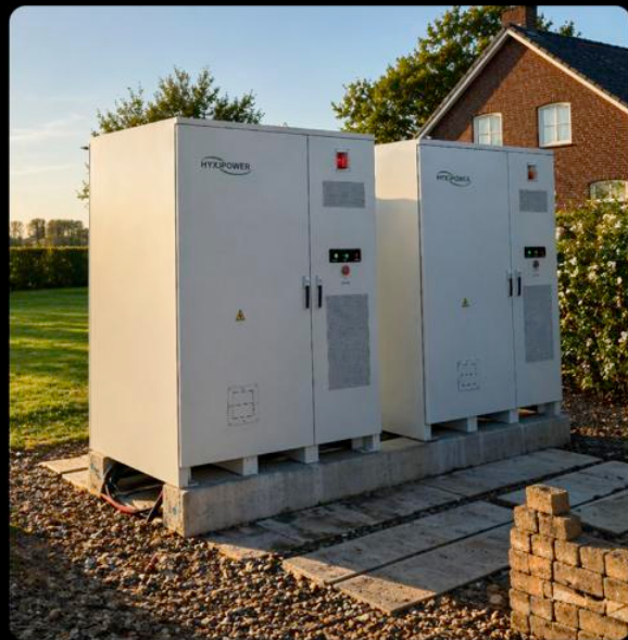
105kW/232kWh C&I ESS Netherlands, Capacity 200kW/430kWh
