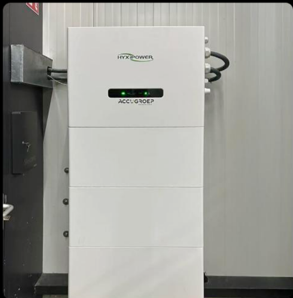
All-in-One ESS Overijssel, Netherlands, Capacity 12kW/20kWh
