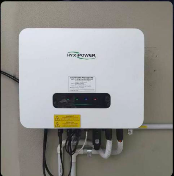
Hybrid Interter Queensland, Australia, Capacity 6.6kW
