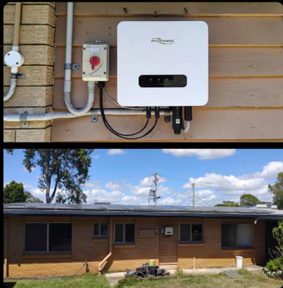
Hybrid Interter Brisbane, Australia, Capacity 6.6kW
