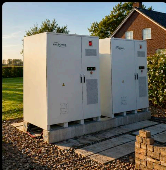
105kW/232kWh C&I ESS Netherlands, Capacity 200kW/430kWh
