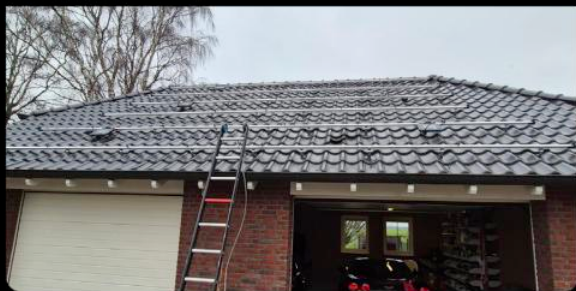
Microinverter Drenthe, Netherlands, Capacity 7.9kW
