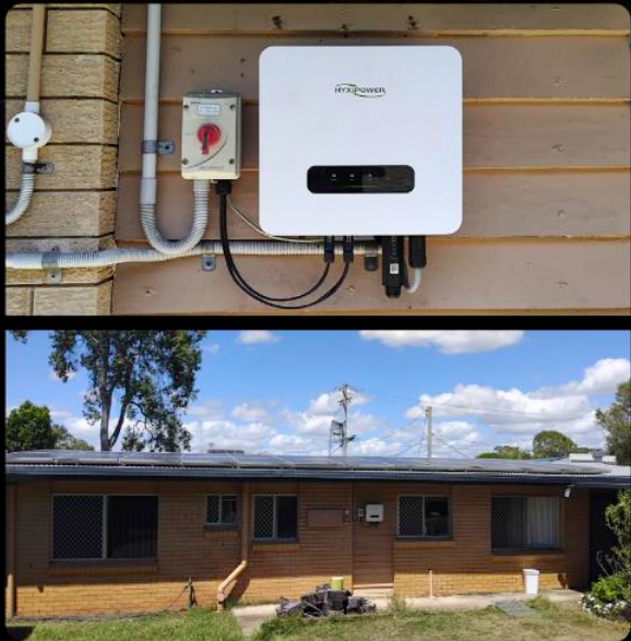
Hybrid Interter Brisbane, Australia, Capacity 6.6kW
