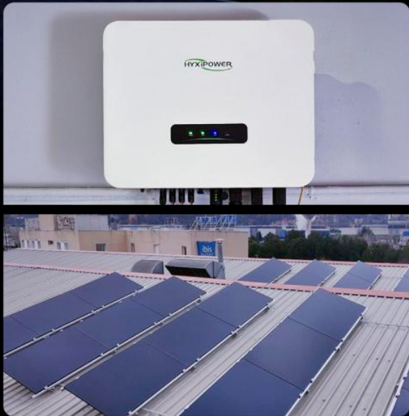
Hybrid Interter Barcelona, Spain, Capacity 25kW
