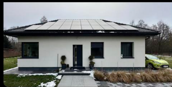
All-in-One ESS Mazovia, Poland, Capacity 10kW
