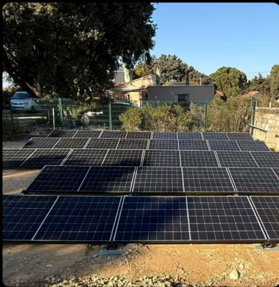
Microinverter Orange, France, Capacity 9kW
