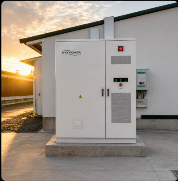
105kW/232kWh C&I ESS Spain, Capacity 100kW/215kWh
