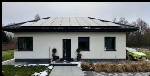
All-in-One ESS Mazovia, Poland, Capacity 10kW
