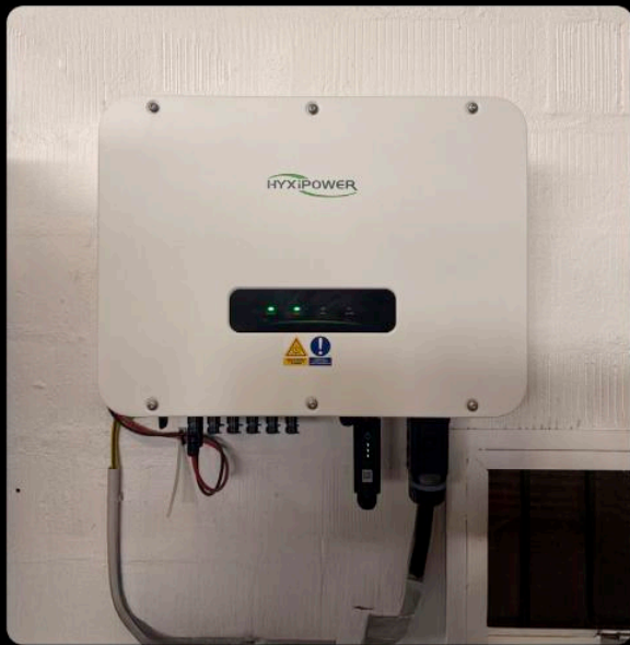
Microinverter Drenthe, Netherlands, Capacity 7.9kW
