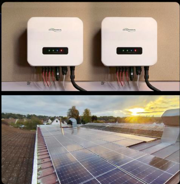
String Inverter Eure-et-Loir, France, Capacity 45kW
