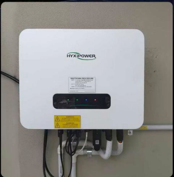
Hybrid Interter Queensland, Australia, Capacity 6.6kW
