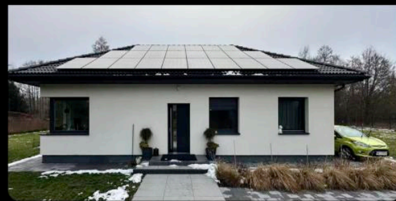
All-in-One ESS Mazovia, Poland, Capacity 10kW
