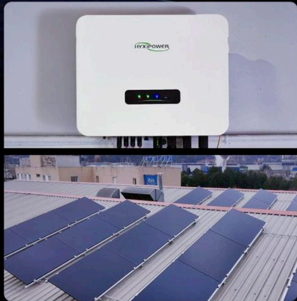
Hybrid Interter Barcelona, Spain, Capacity 25kW
