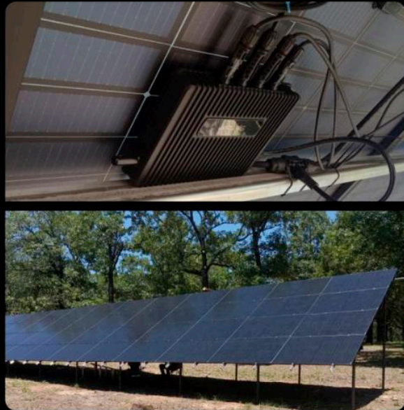
Microinverter Arkansas, USA, Capacity 11.6kW
