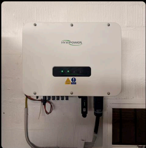
Microinverter Drenthe, Netherlands, Capacity 7.9kW
