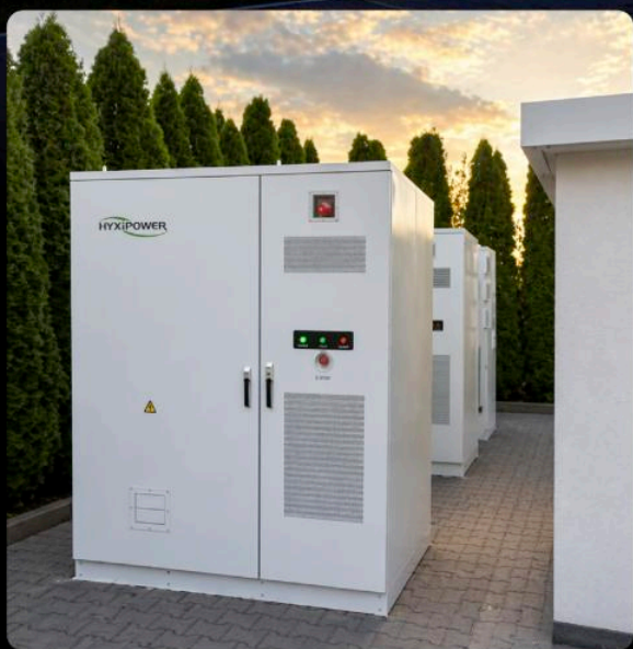
100kW/215kWh C&I ESS Poland, Capacity 200kW/430kWh
