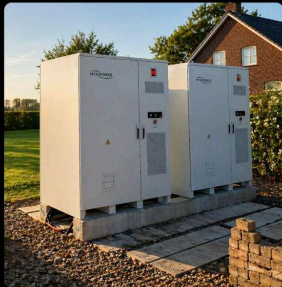
105kW/232kWh C&I ESS Netherlands, Capacity 200kW/430kWh
