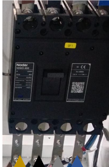
Uu Uv Uw N From grid side
