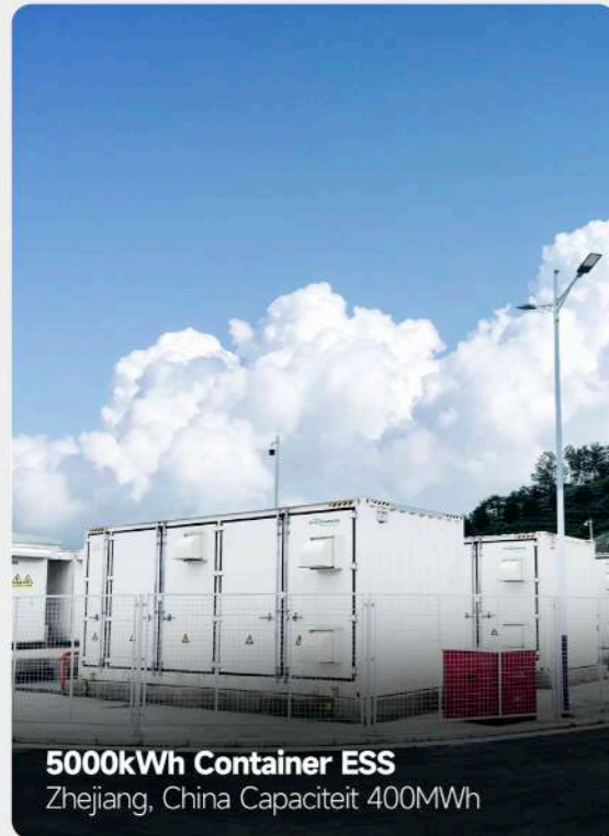
5000kWh Container ESS Zhejiang, China Capaciteit 5MW/10MWh
