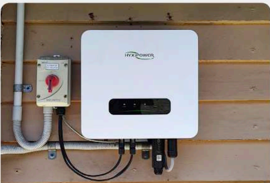
String Inverter Eure-et-Loir, France Capacity 45kW
