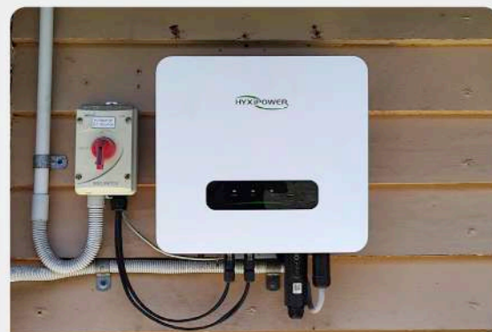
String Inverter Eure-et-Loir, France Capacity 45kW
