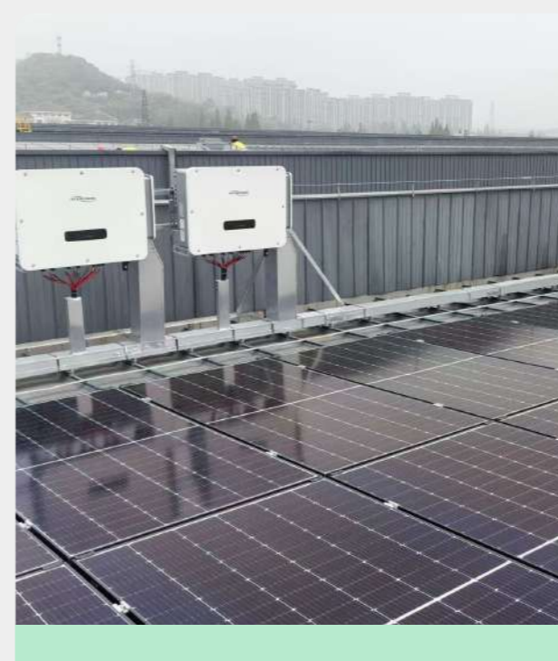
50kW/110kW String Inverter Zhejiang, China Capacity 4MWp
