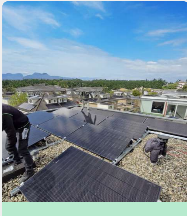
Hybrid Inverter, High Voltage Battery Rotterdam, Netherlands Capacity 10kW
