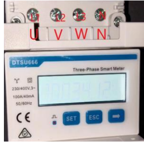
Wiring Diagram (Top Side of Electricity Meter)
