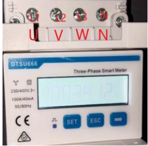
Wiring Diagram (Top Side of Electricity Meter)
